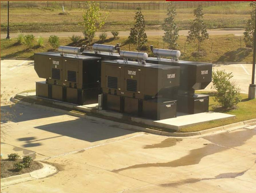
Full Operational Emergency Back Up is powered by four 400 KVA diesel generators. These power units will prevent company and employee down time during events that interrupt the main power supply from the utility supplier.
